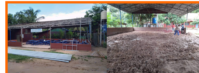
Bakong's cafeteria received a new tile floor and roof!
